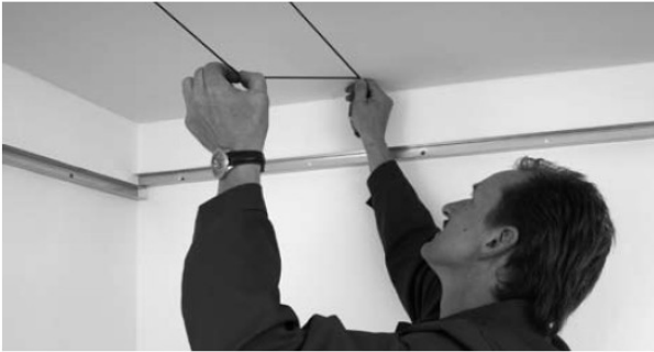
Applying the ceiling grid.
