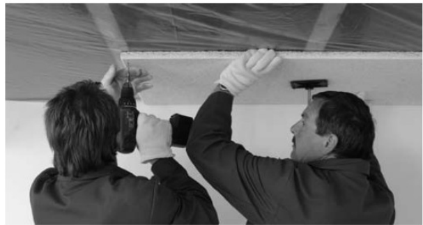
Installing the panels by means of supports. Press the panel onto the lath with the ball of the hand while screwing. There mustn't be a gap between the panel and the wood lath. Only work with the panels with clean hands and a clean tool.
