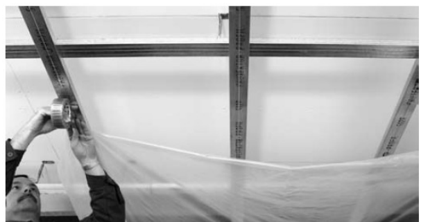
Alternative: Insertion of PE sheeting as trickle protection or a vapour barrier matching the installation of the Heradesign panels. Stick sheet joints together.
