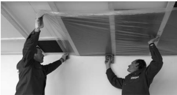
Alternative: Insertion of PE sheeting as trickle protection or a vapour barrier matching the installation of the Heradesign decorative panels. Stick sheet joints together.
