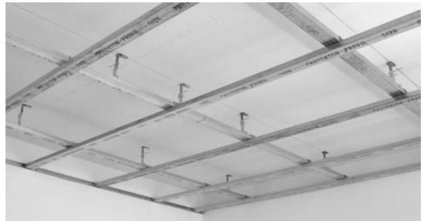
Finished ceiling grid.
