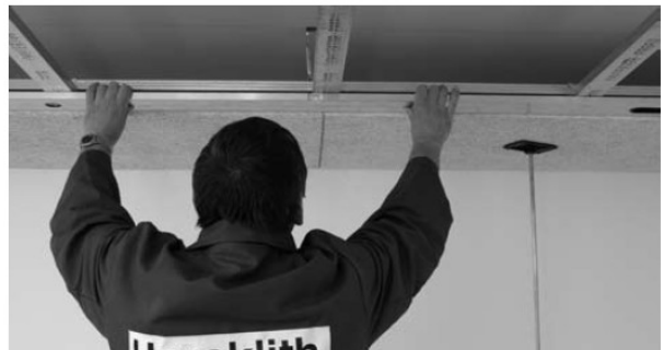
Align the panel rows with an installation lath. Panel joints must be positioned to be centred under the section. No free, suspended panel joints are allowed.
