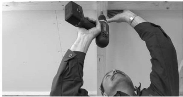
Installation of the main joists and cross joists.
