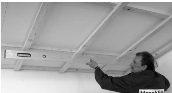
Aligning the laths with a spirit level or laser level.
