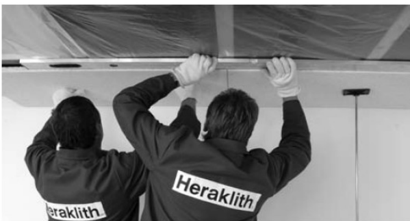
Align the panel rows with an installation lath. Panel joints must be positioned to be centred under the section. No free panel joints are allowed.
