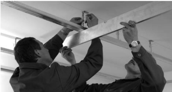
Aligning the CD sections with a spirit level or laser level.
