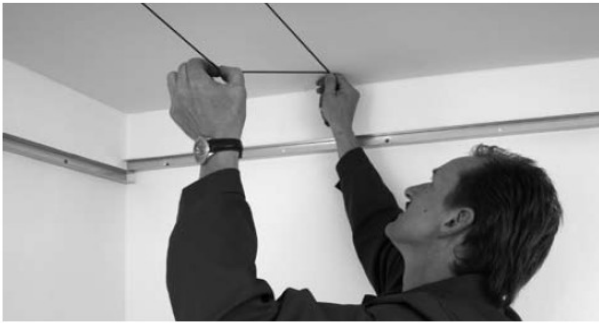
Applying the ceiling grid from the centre of the room, e.g. by using a chalk line. Pay attention to having equal sized edge fields at the sides of the room.
